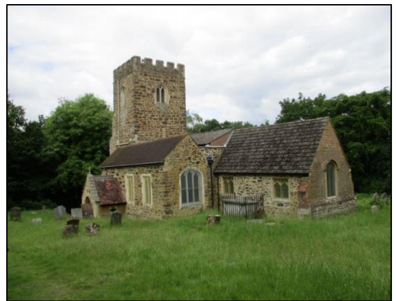
Retiling & repair of s porch
