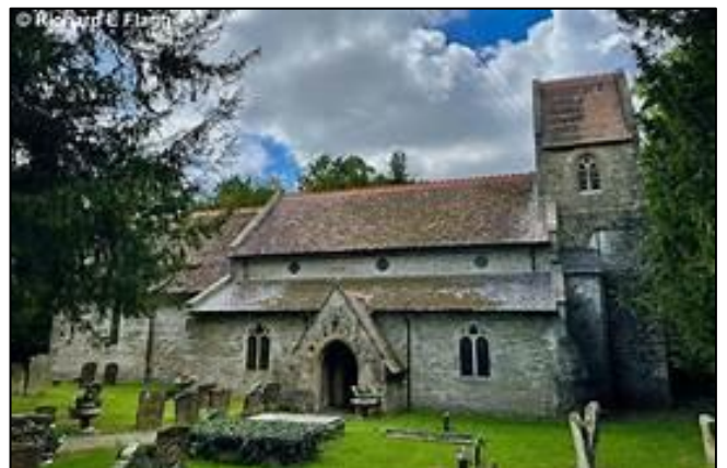
Clearance of bio waste from church tower and installation of bird protection grilles
