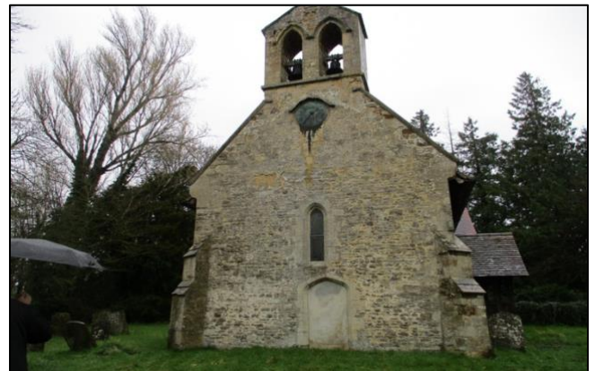
Steel pinning of north wall and associated groundworks and archaeology
