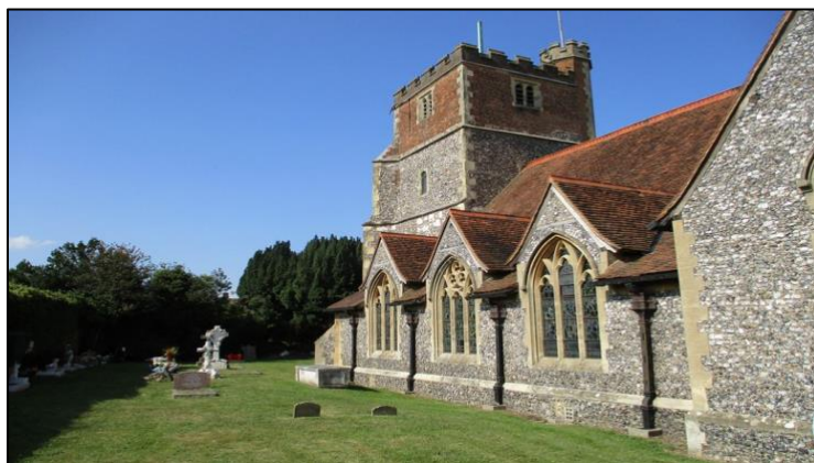
Repairs to the east end of the church including Lady Chapel plinth, repointing in south wall and repairs to the SW buttress to tower
