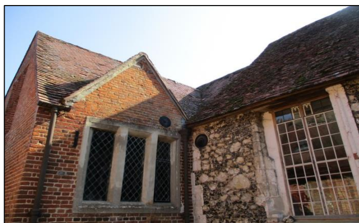
Stripping and retiling of the chapel roof and the north slope of the chancel
